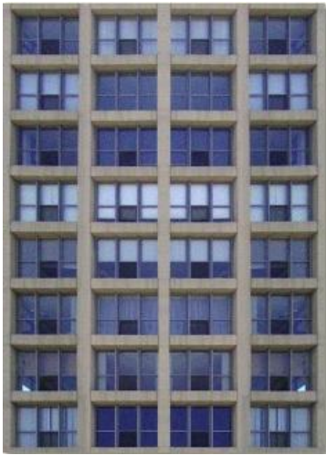
Figure 10: Input image of a façade
